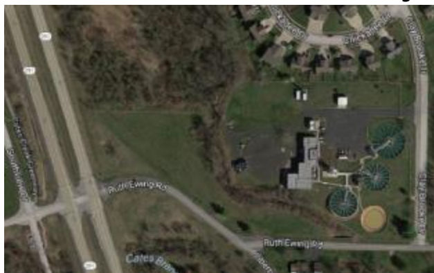
Water Treatment Plant – Training Location
